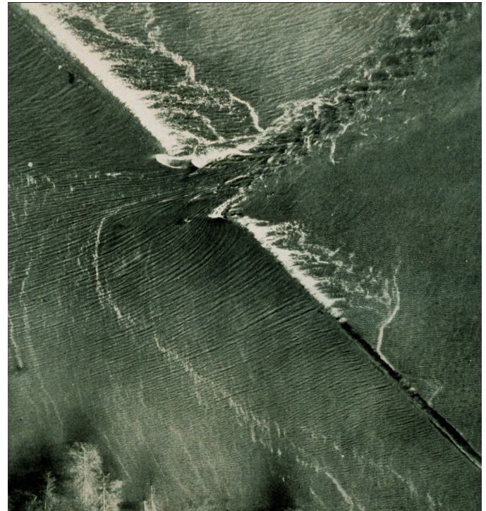
Figure 1: April 1927 Flood of the Mississippi River, levee break, Greenville Mississippi, US. National Oceanic Atmospheric Administration
